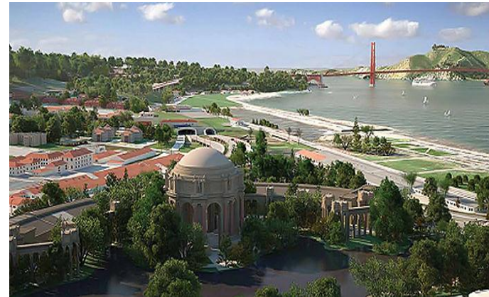
Presidio Parkway Project, San Francisco, California, USA
